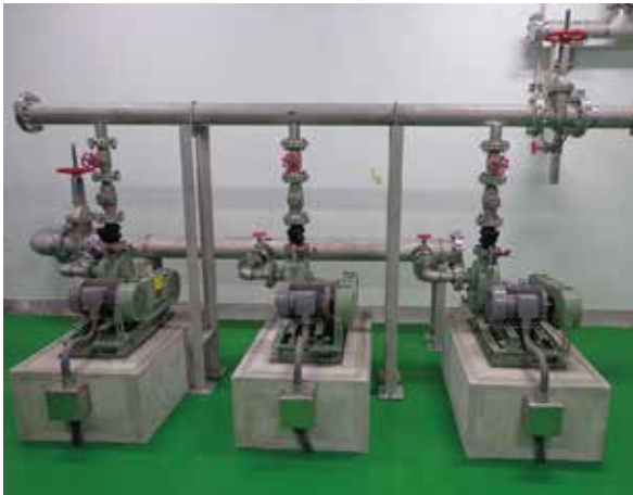
農業集落排水処理施設 汚泥引抜ポンプ Residential wastewater treatment facility Sludge withdrawal pump
